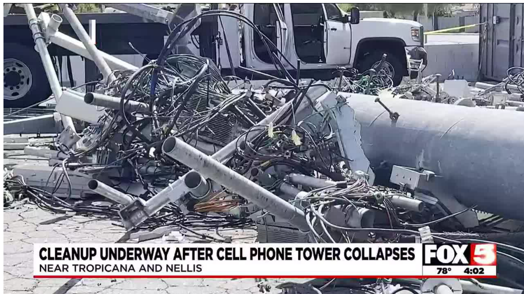
Visual Image courtesy of FOX 5 Las Vegas, used for informational purposes under fair use – The image demonstrates the structural safety risk of cell towers.
