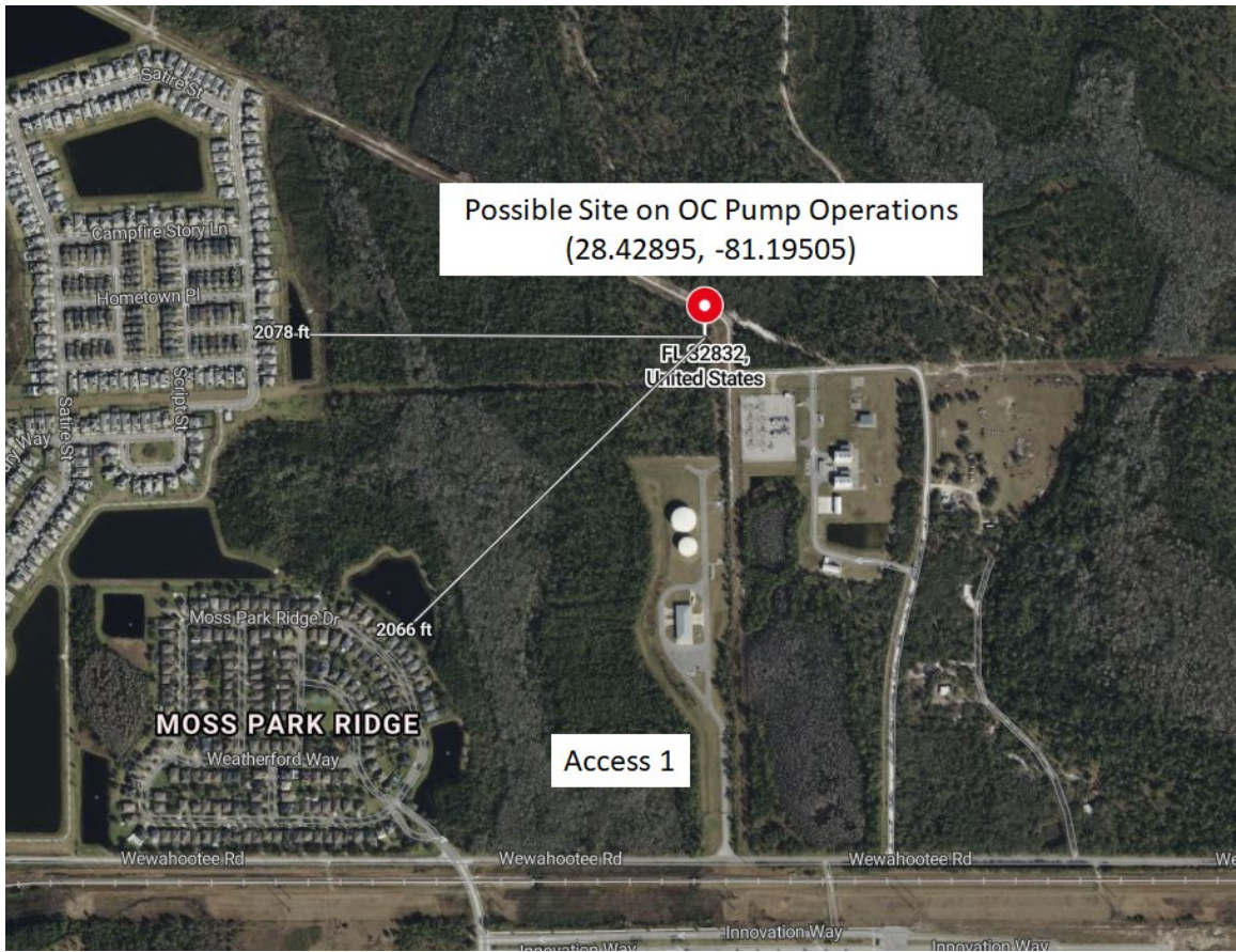
The Orange County Pump Station (Visual Aid Identifier 4) is located over 2,000 feet from the nearest residences, offering an ideal buffer zone while supporting infrastructure needs
