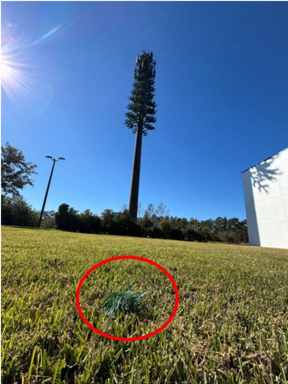
Fallen faux foliage from a cell tower at 8553 Commodity Circle, Orlando, FL 32819 – Site 2, fallen Foliage atop recently cut turf to the East of the tower. This image underscores the environmental concerns posed by synthetic materials degrading and dispersing into nearby ecosystems, including wetlands and residential areas.
