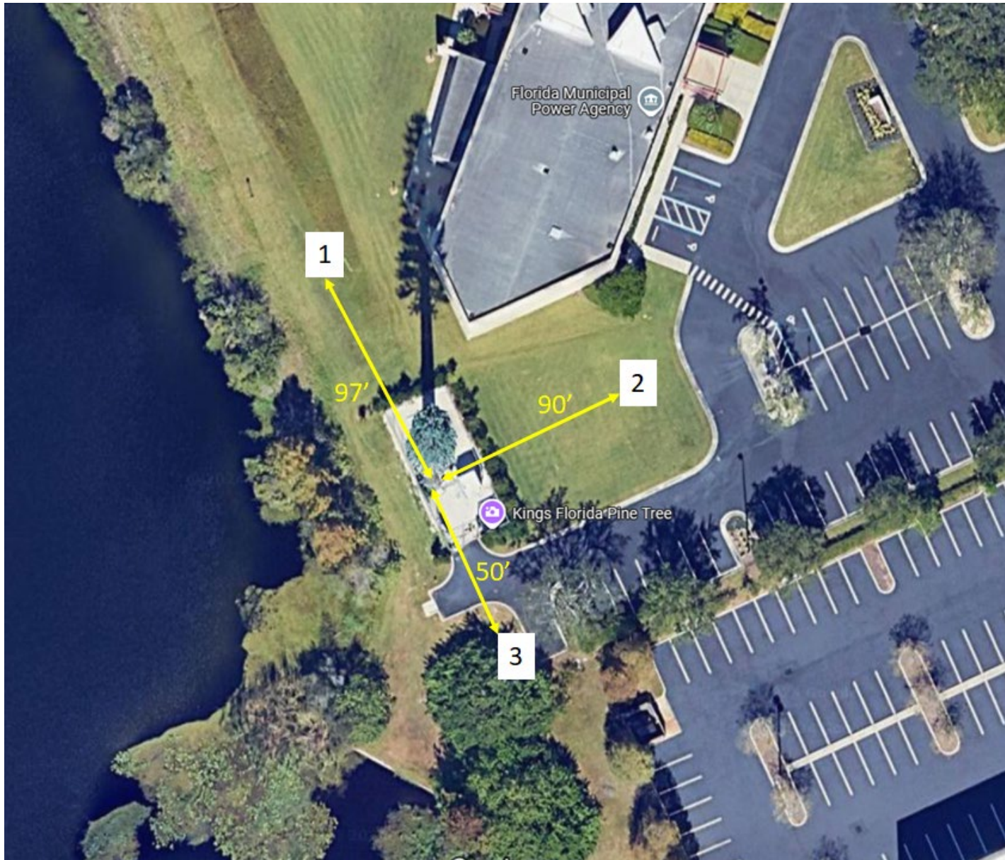
Fallen faux foliage from a cell tower at 8553 Commodity Circle, Orlando, FL 32819 – Fallen Foliage locations and estimated distance from tower.
